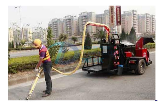
Crack sealing machine
